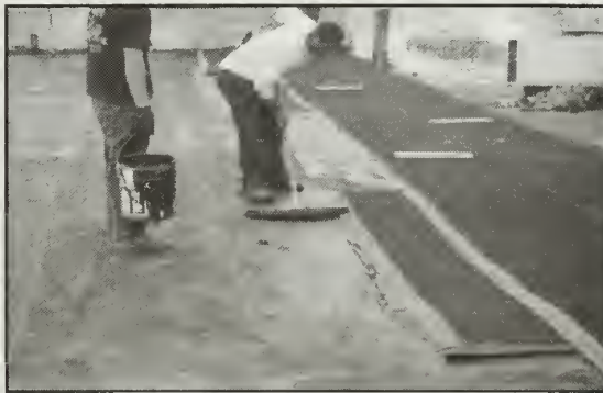
Below: (L) .040 aluminum edge was installed (R) Rubberized black granule modified bitumen cap sheet was installed over two base piles
